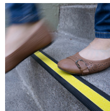
Exterior Cement Stairs
